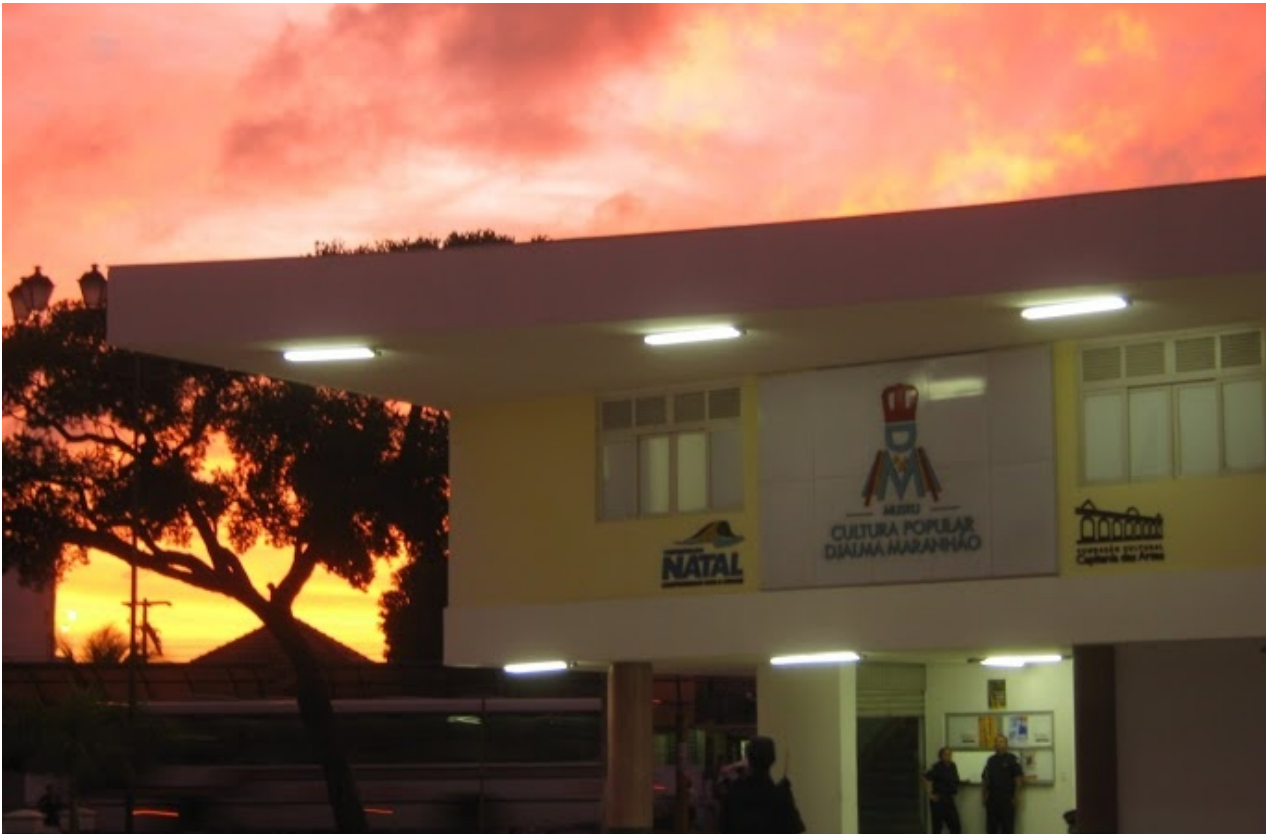
The place where the workshop happened during one week.
